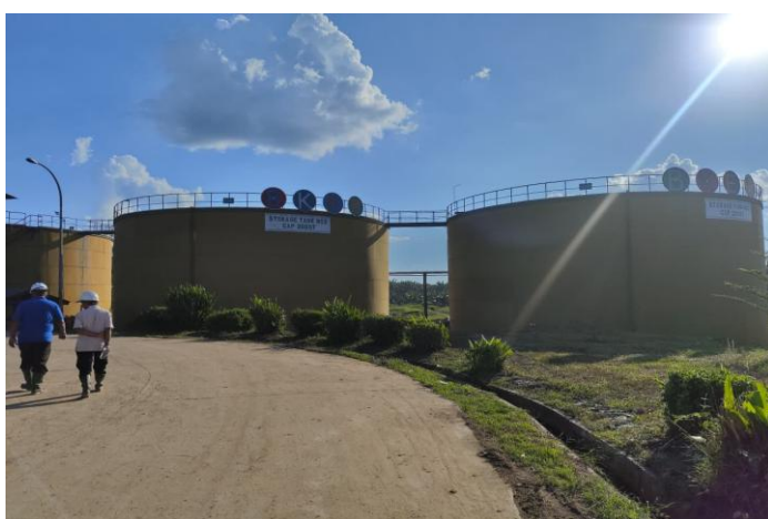
Figure 15. CPO Mill Storage Tank
