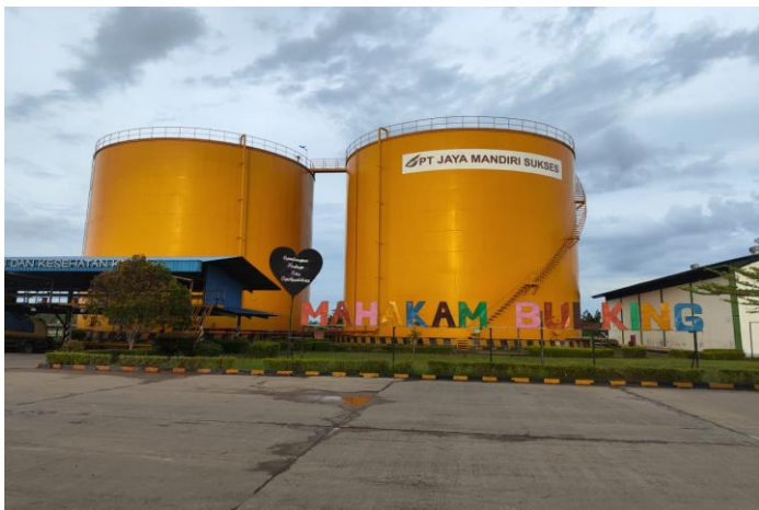
Figure 1. CPO Storage Tank
